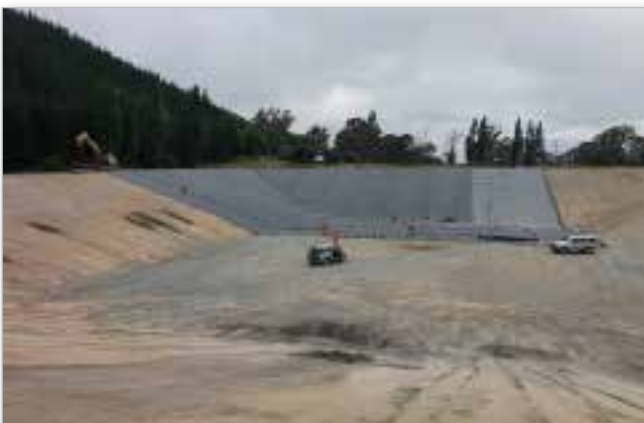
Vineyard dam being lined
